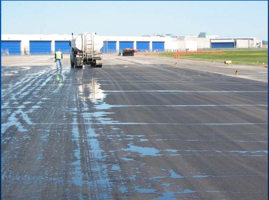
**Water testing for slope verification**
