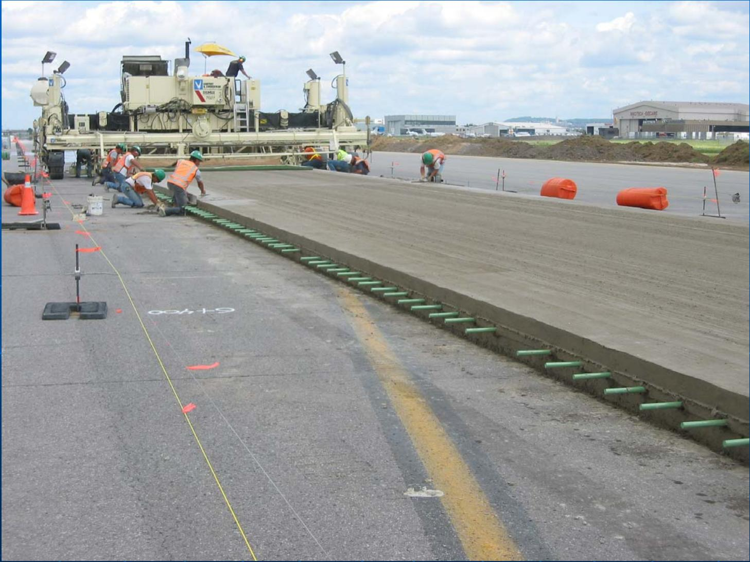
**Dowels installation during paving**
