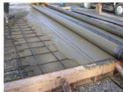
Photo 2: Concrete consistency and rebar facilitate build-up of concrete to top of formwork.
