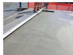
Photo 5: Application of broom texture finish.
