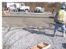
Photo 3: Concrete consistency past extent of rebar is self-leveling.
