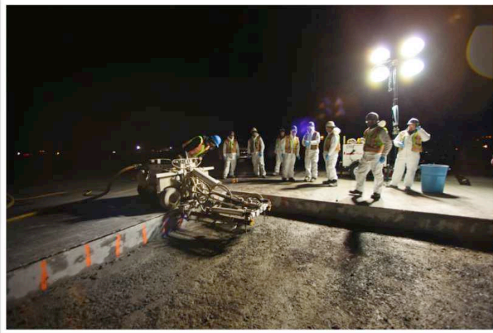
Time 21:40 – 02:00 • (Area A) • Gang-drilling PCC for Dowel Placement (30mins Ahead of Schedule)
