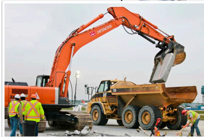
Time 20:35 • (Area A) • Removal of 2.5m x 2.0m PCC Slabs with 2 nd Excavator
