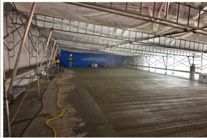
Time 05:30 • (Area A) • Wet Curing at 20-25°C (On Schedule)
