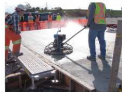
Photo 4: Power trowel with pan float and fog misting of the concrete surface.
