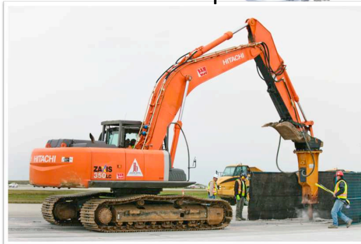
Time 20:10 • (Area A) • PCC Demolition with Hydraulic Hammer
