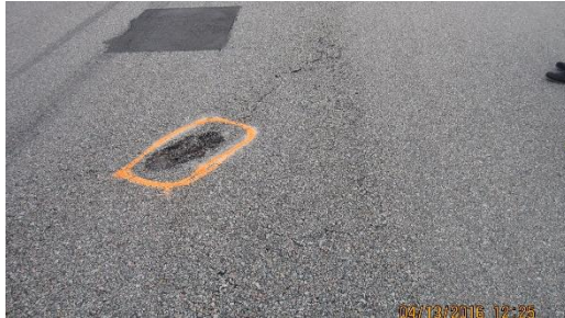
Raveling; interconnected fine cracks near 13-31
