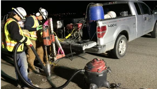
Obtaining initial cores, June 2016
