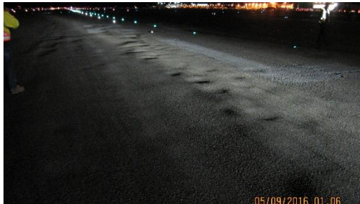
Tire “dimpling”, rutting, shoving, south side of centreline near 26L
