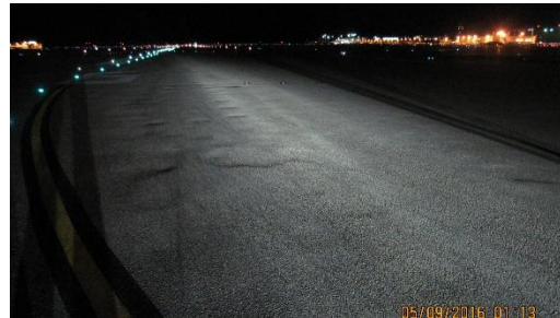
Tire “dimpling”, rutting, shoving, north side of centreline near 26L
