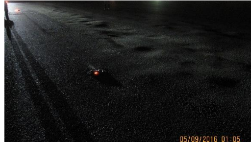
Tire “dimpling”, rutting, shoving on centreline near 26L
