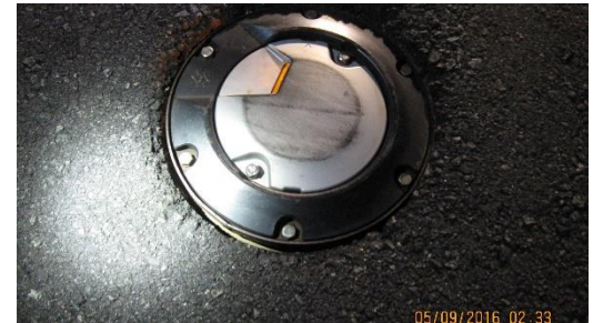
Inset light, missing perimeter sealer, perimeter raveled
