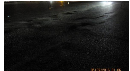
Tire “dimpling”, rutting, shoving, south side of centreline near 26L
