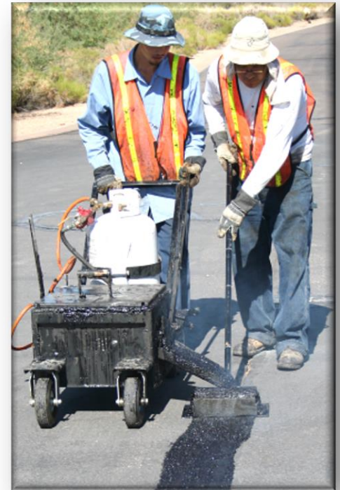
Using a material handler
