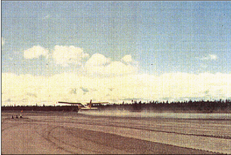
Gravel Surface - Dust Generation
