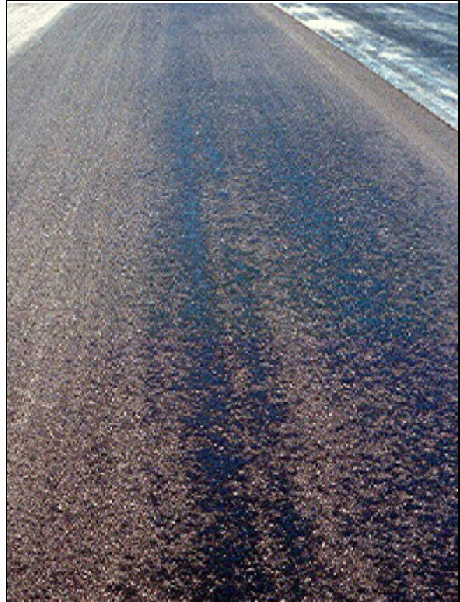
Bleeding Low to Medium Severity
