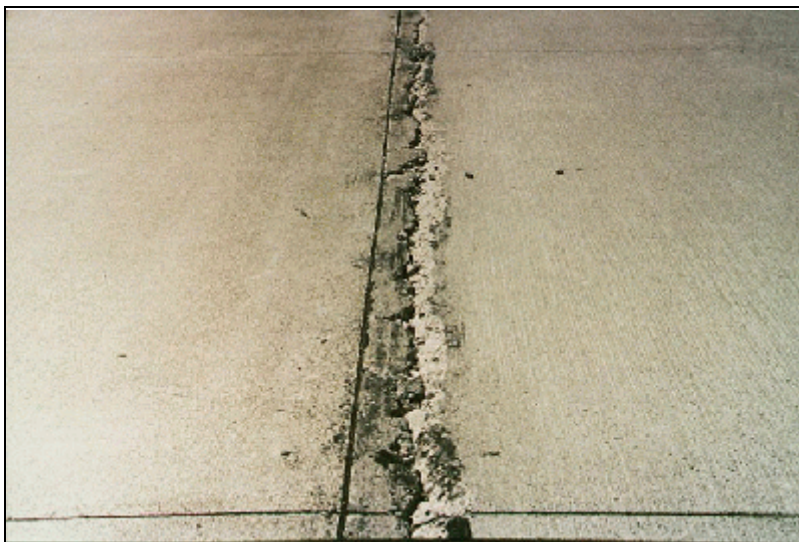
Edge Cracking - High Severity
