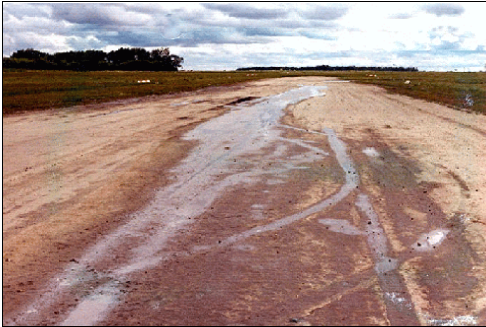
Gravel Surface - Poor Drainage Due to Loss of Crown
