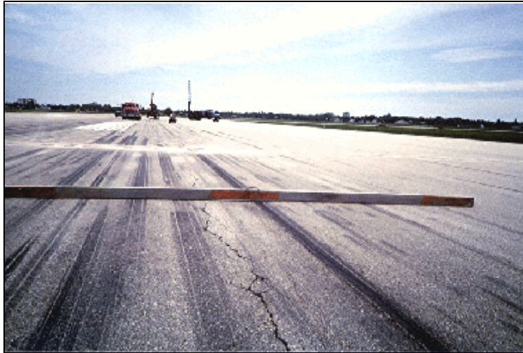
Rutting - Low Severity
