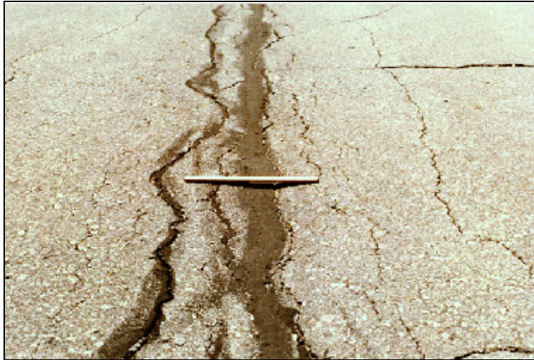
Transverse Crack - High Severity
