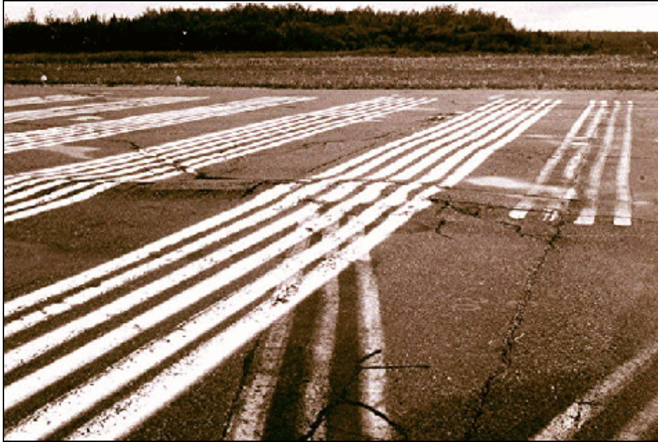
Frost Heaving - Major Severity
