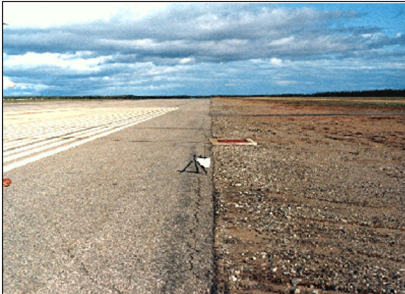
Edge Cracking - Low Severity
