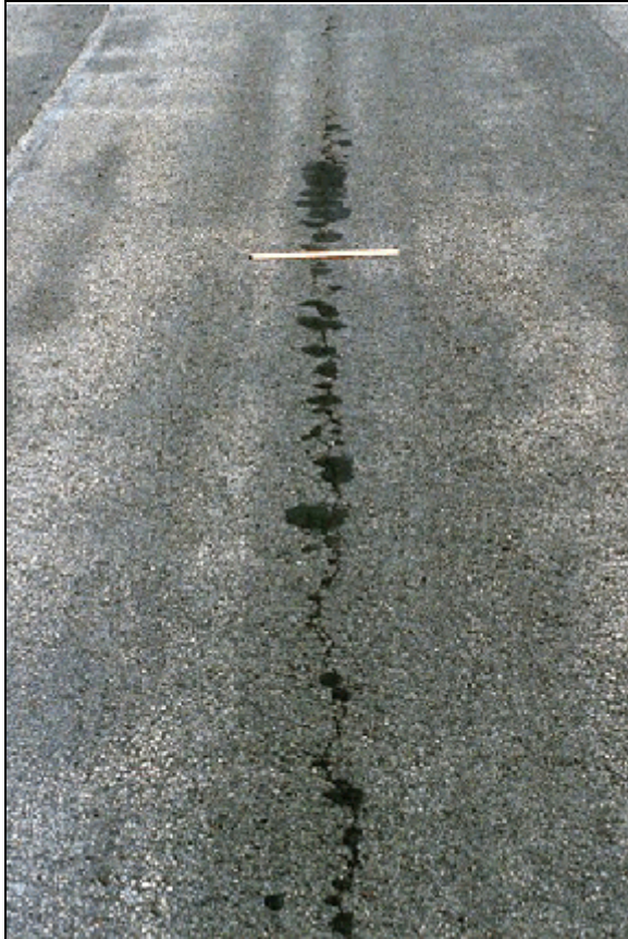
Bleeding - Low Severity (Bleeding of Crack Sealant Through the Overlay)
