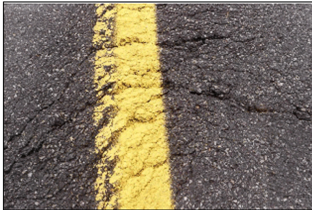
Distortion - Low to Medium Severity
