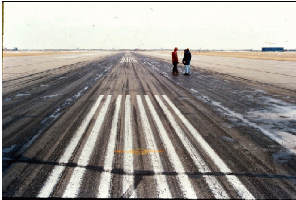
Rubber Deposits - Low to Medium Severity
