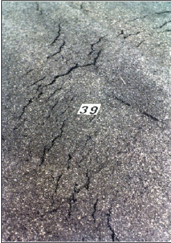
Tear Cracking - Low to Medium Severity
