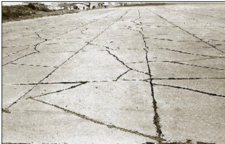
Panel Cracking - Medium to High Severity
