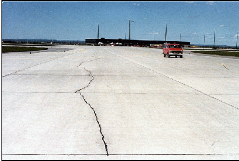
Panel Cracking - Low Severity
