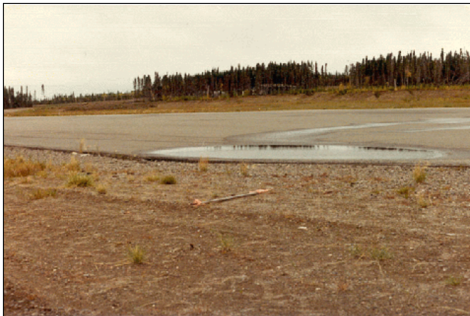
Subgrade Settlement - High Severity
