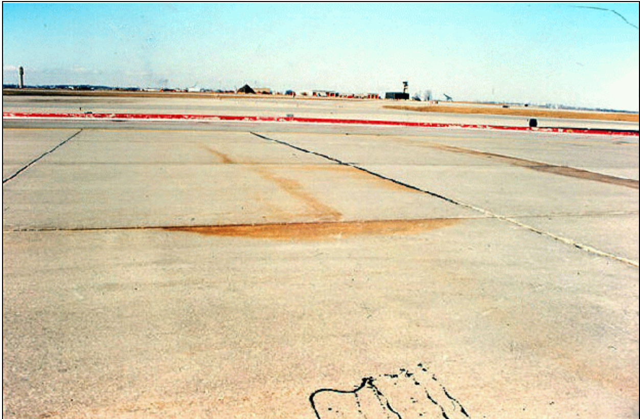
Concrete Slab Pumping (Evidenced by Surface Staining at the Joints)
