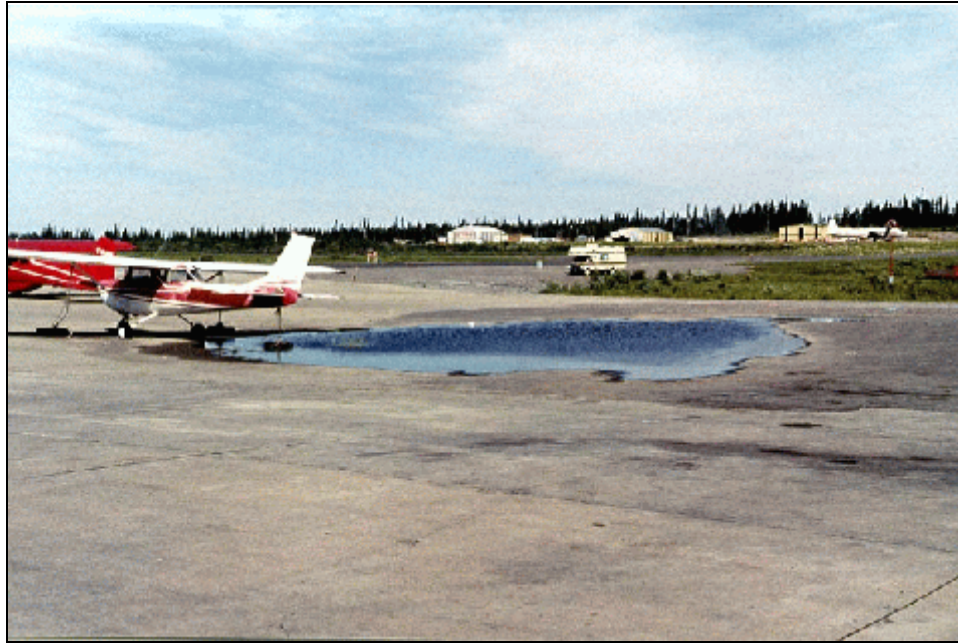
Subgrade Settlement - High Severity (Due to Permafrost Degradation)
