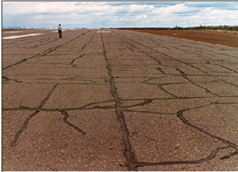
Block Cracking - Low Severity
