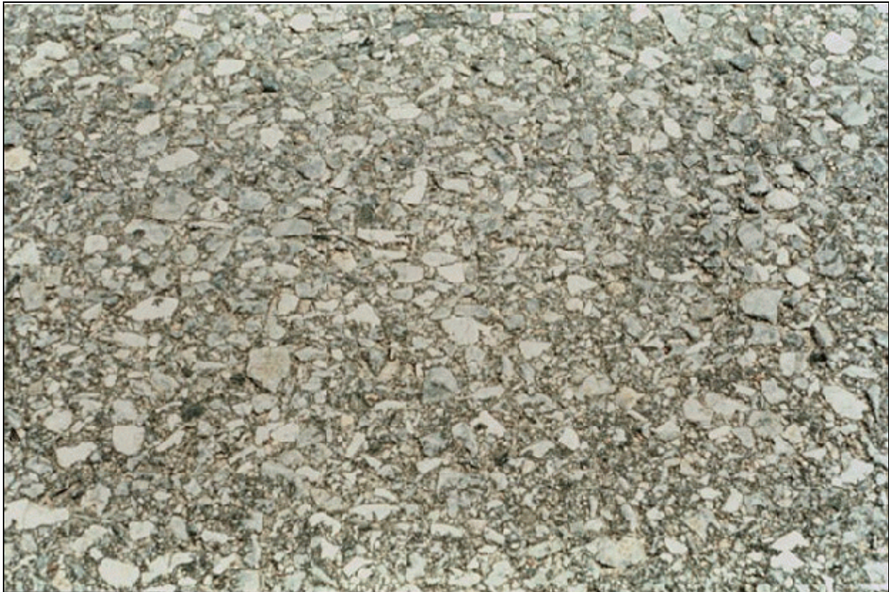
Wear and Polish - Low to Medium Severity
