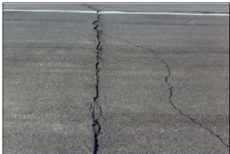
Transverse Crack - Medium Severity
