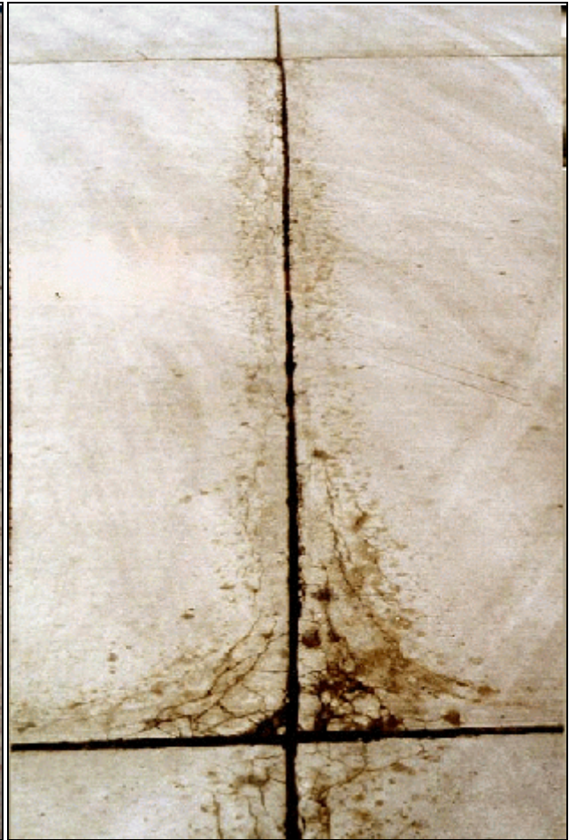
"D" Cracking (Characteristic Curve Pattern Around Slab Corners)
