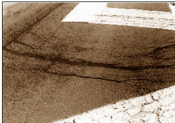
Distortion - Medium to High Severity
