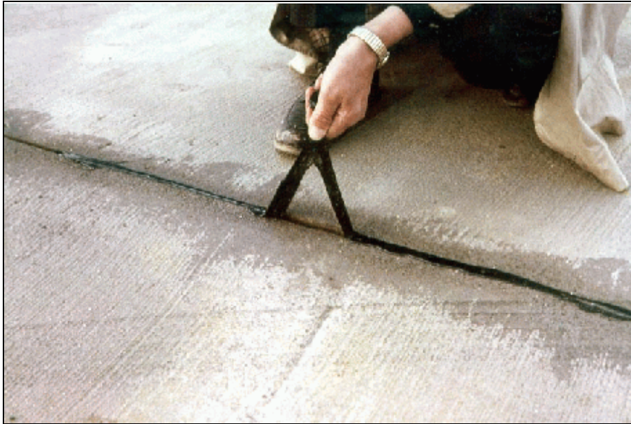
Joint Sealant Failure - Medium Severity (Sealant Adhesion Loss on Both Sides)
