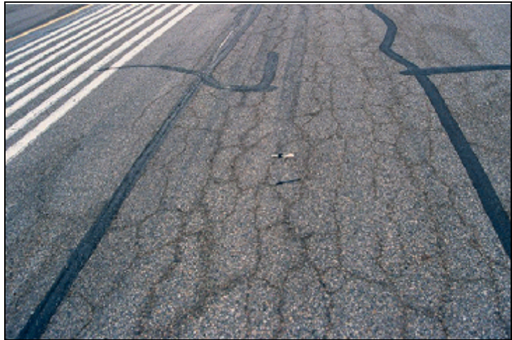
Alligator Cracking - Medium Severity
