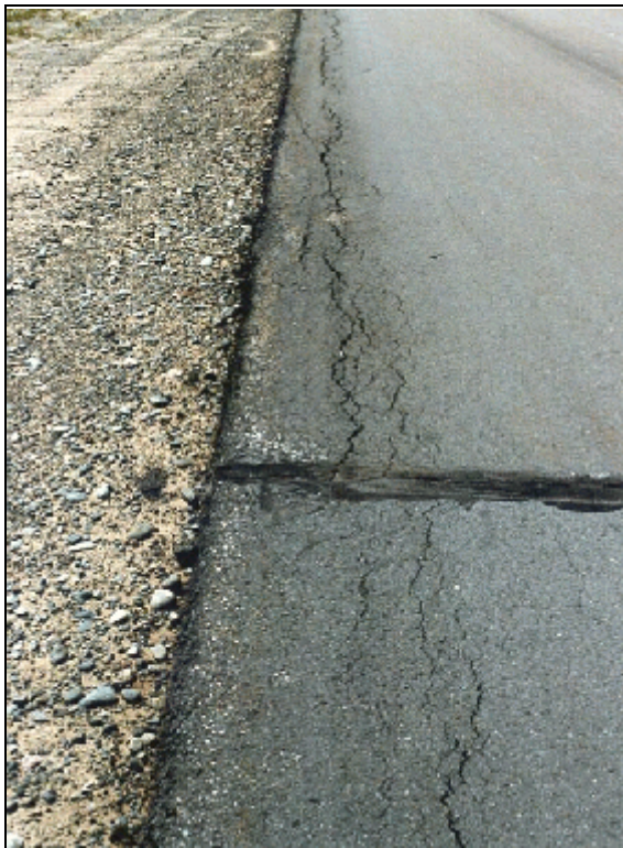
Edge Cracking - Medium Severity
