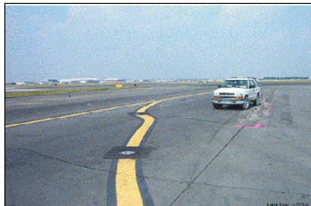
Distortion - High Severity (Without Associated Tear Cracking)
