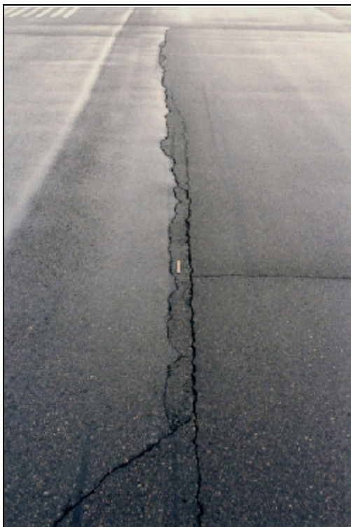
Longitudinal Crack - Medium Severity
