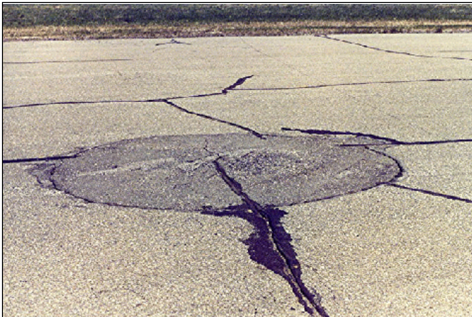
Frost Heaving - Subgrade Boulder Being Raised
