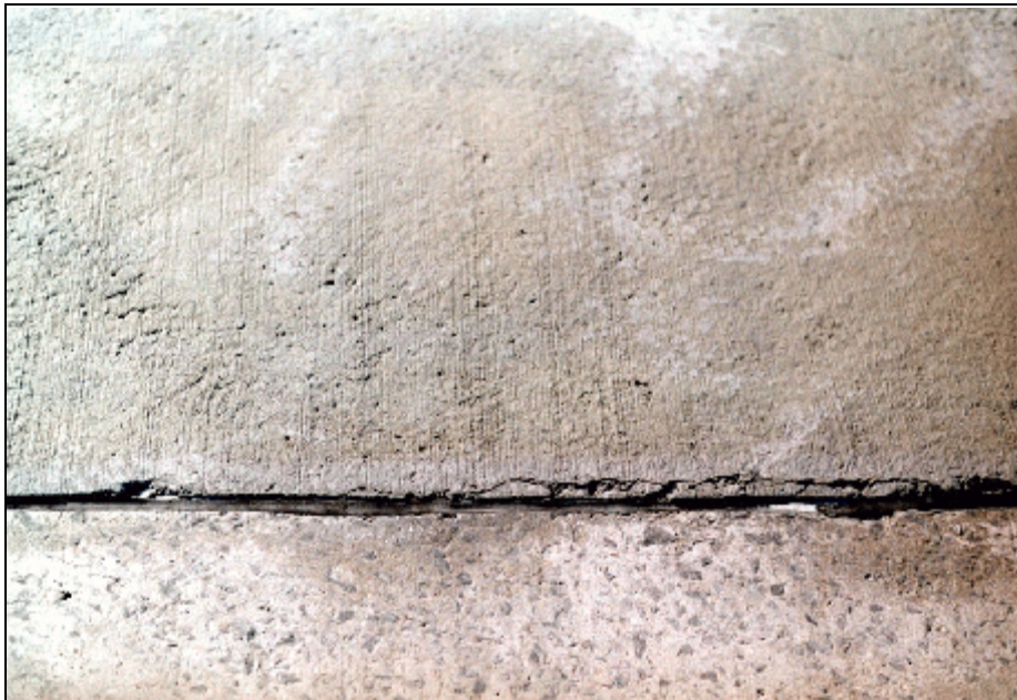
Joint Sealant Failure - High Severity (Joint Edge Chipping)
