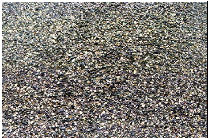
Ravelling - Medium Severity
