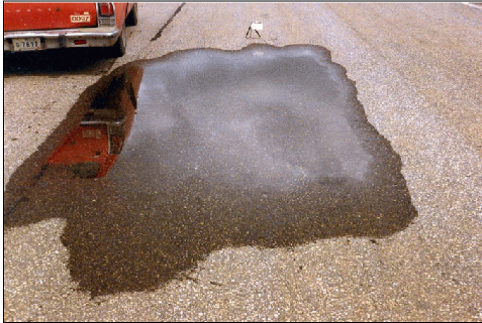
Bird Bath - Medium Severity
