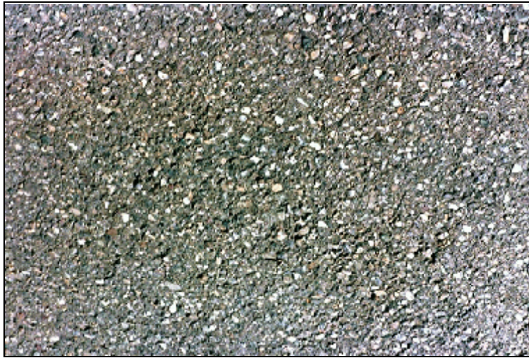
Ravelling - Low Severity
