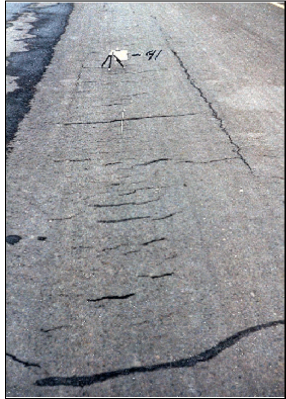
Tear Cracking - Medium Severity
