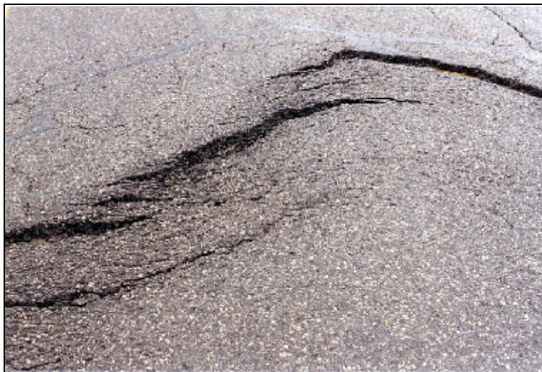
Tear Cracking - High Severity
