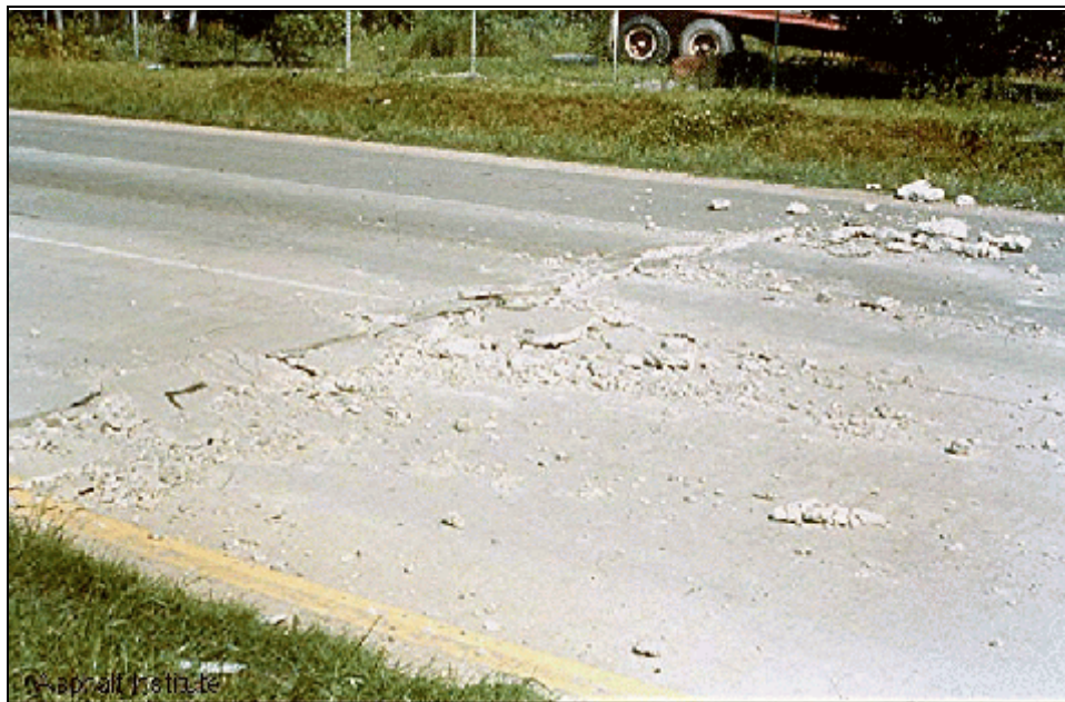
Compression Buckling
