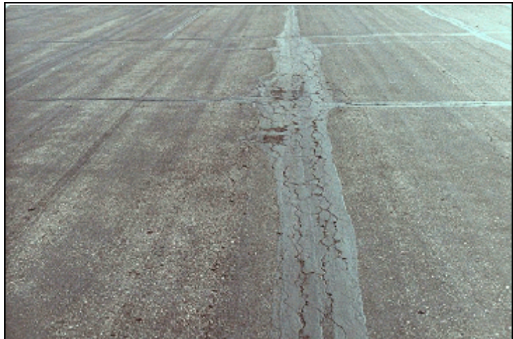
Longitudinal Crack - High Severity
