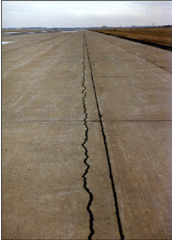
Edge Cracking - Low Severity
