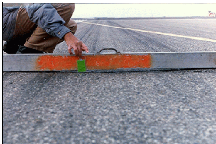
Rutting - Medium Severity
