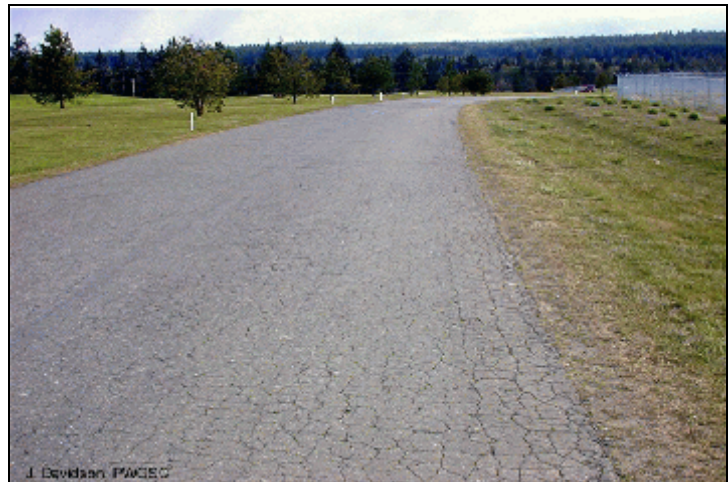
Block Cracking - High Severity (May Look Like Alligator Cracking But Is Not Limited to the Wheelpath Area)
