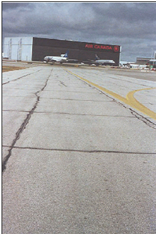
Reflection Cracking (Cracks Reflected from Joints in the Underlying Concrete Slab)
