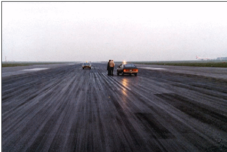
Rubber Deposits - High Severity
