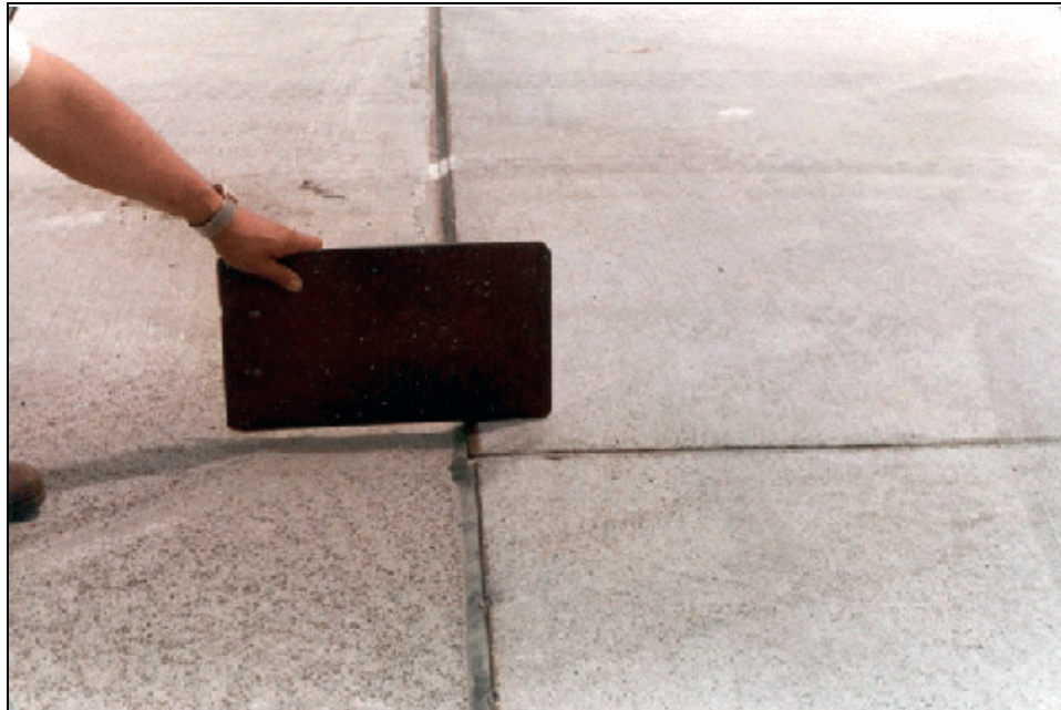
Joint Faulting - Medium Severity
