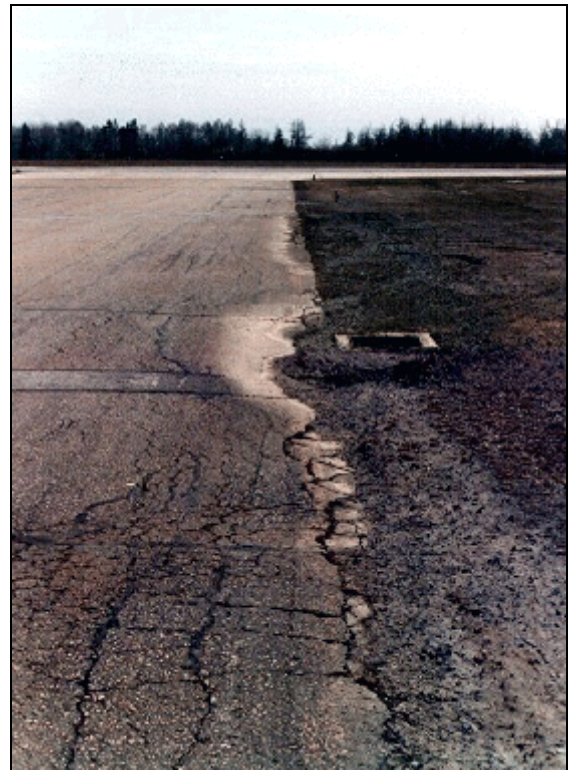
Edge Cracking - High Severity
