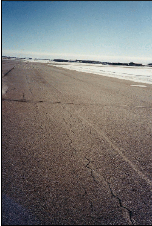
Alligator Cracking - Low Severity (Longitudinal Cracks Appear Initially - Transverse Cracks to Complete the Alligator Pattern Will Soon Follow)
