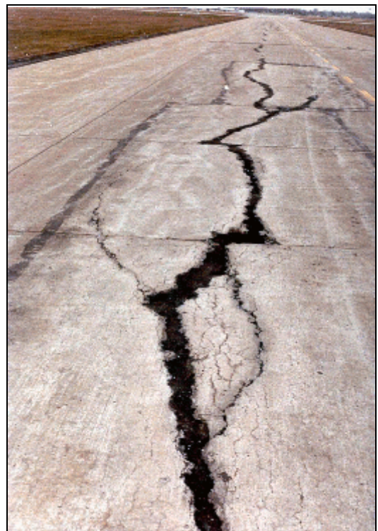
Panel Cracking - High Severity
