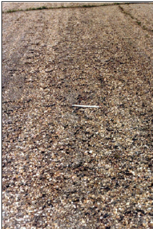
Ravelling - High Severity
