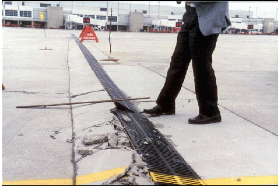
Compression Buckling at an Inserted Surface Drainage Line
