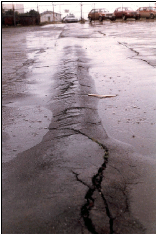
Rutting - High Severity
