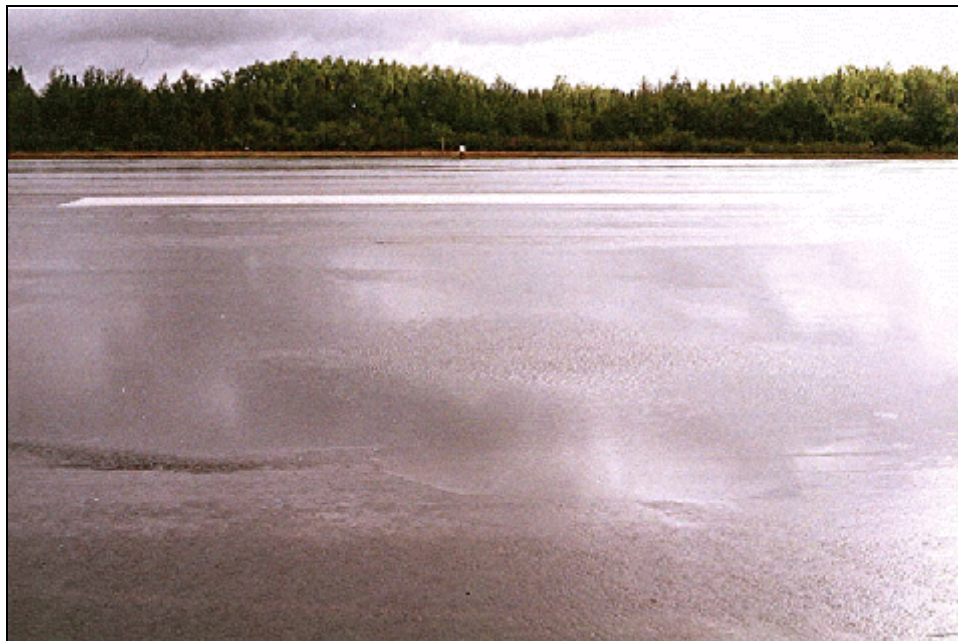
Bird Bath - High Severity
