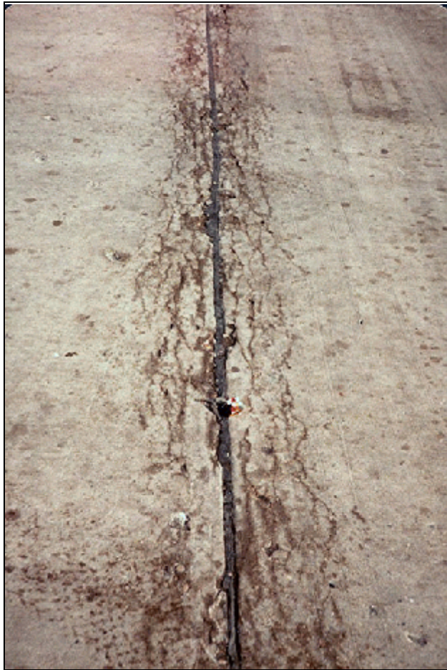
"D" Cracking Medium to High Severity
