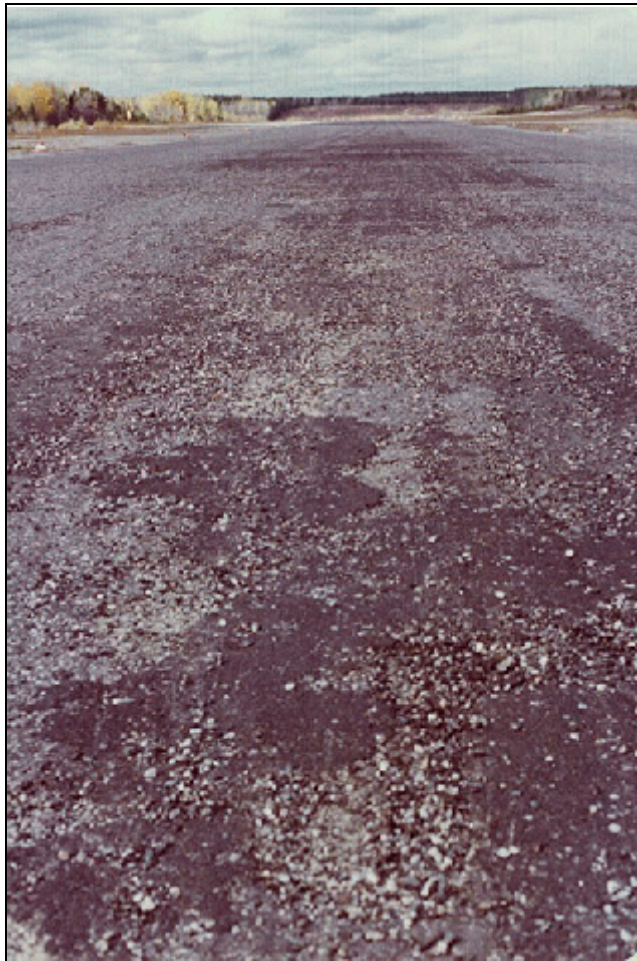
Gravel Surface - Heavily Oiled
