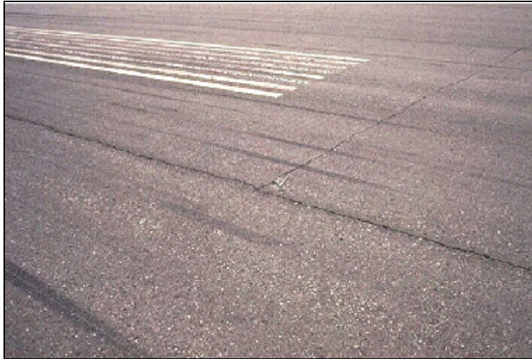
Transverse and Longitudinal Cracking - Low Severity
