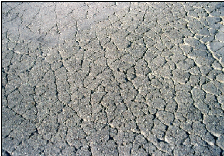
Alligator Cracking - High Severity
