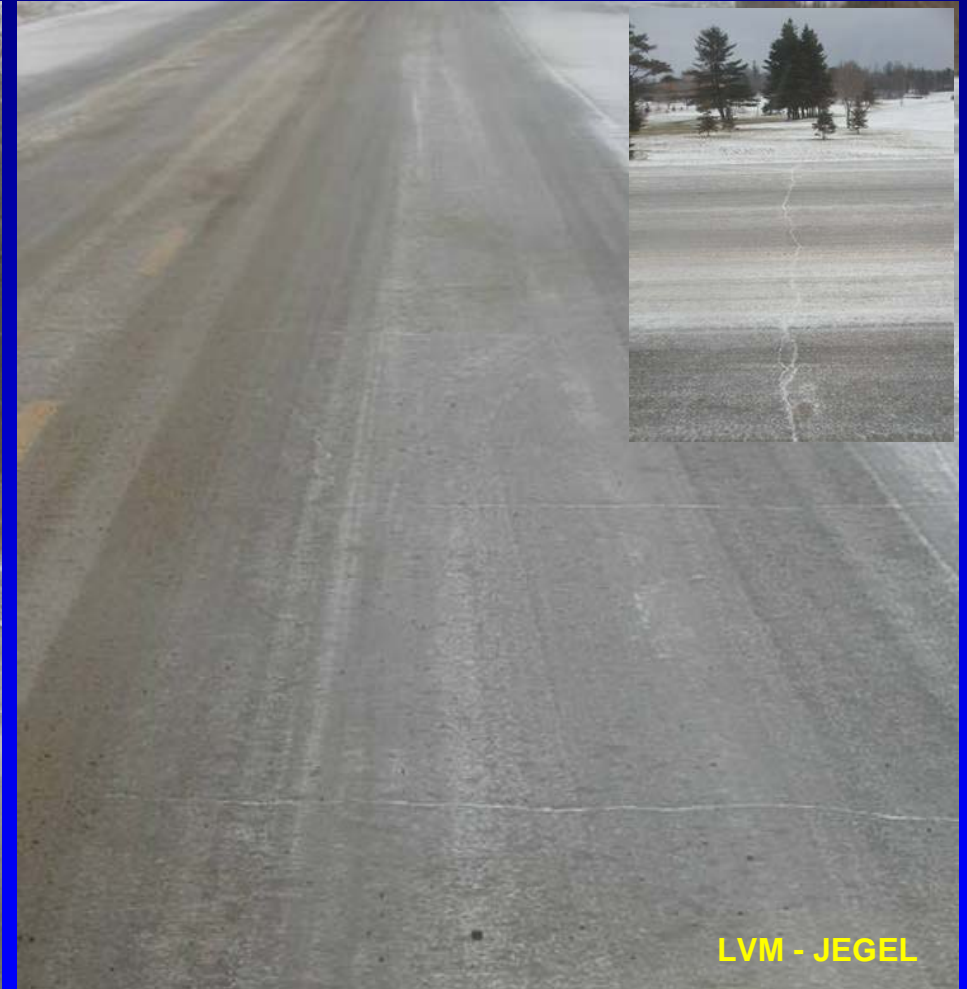
CONDITION OF ADJACENT 1997 MILL/HMA OVERLAY WITHOUT CIR – SIGNIFICANT CRACKING
