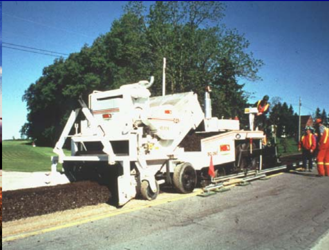
PROCESSED RECYCLED MATERIAL PLACED WITH PAVER
