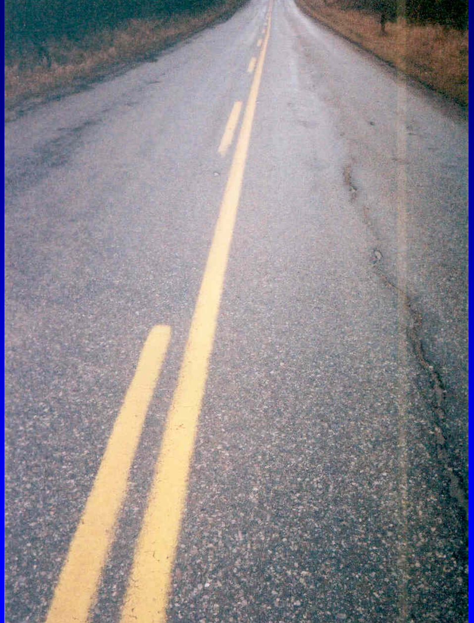
WR 50 CONDITION IN JANUARY 2007 NOTE DISTRESS IN POOR DRAINAGE AREA
