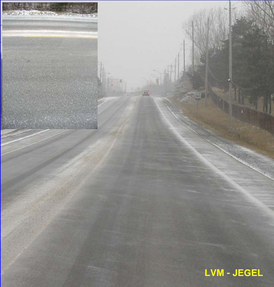
CONDITION OF SUPERPAVE HMA IN 2004 NO CRACKING
