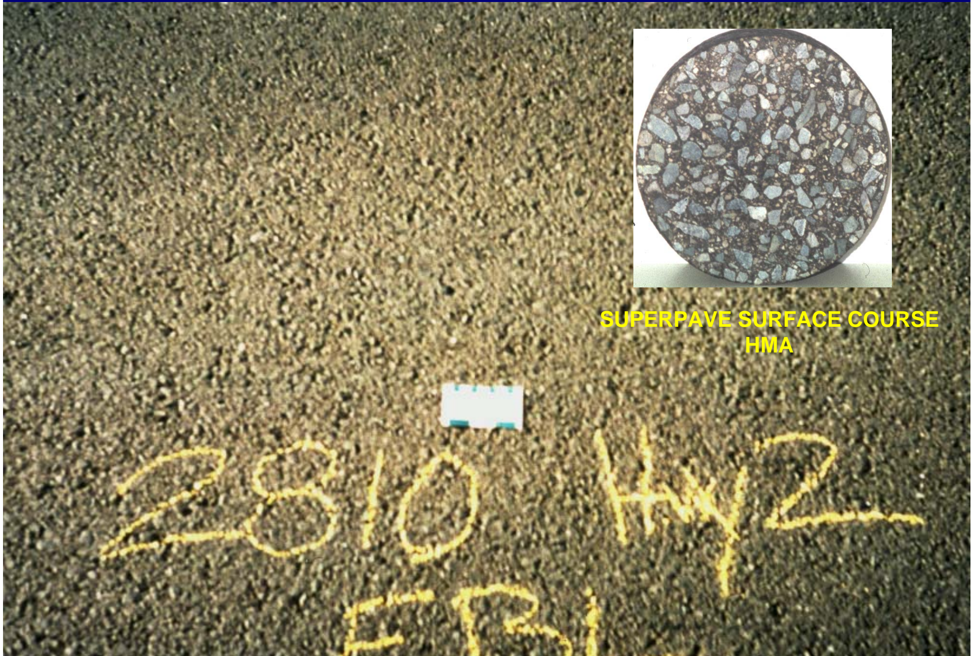
TEXTURE OF SUPERPAVE SURFACE COURSE (~MODIFIED HL1)
