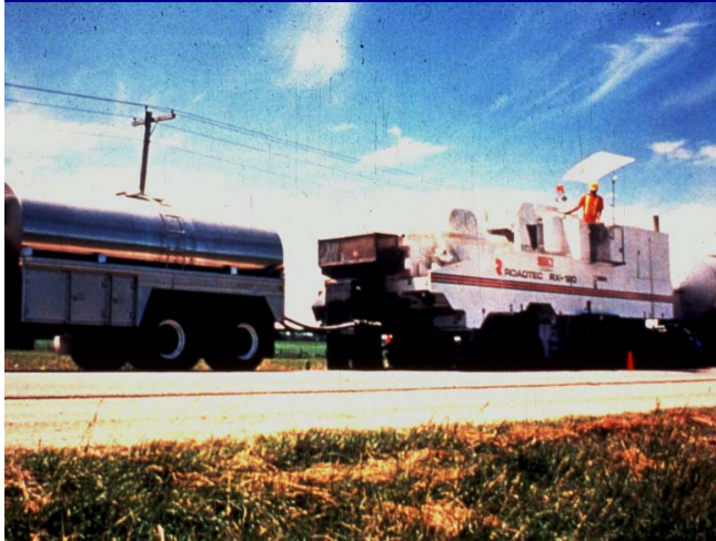
PAVEMENT MILLED/SIZED AND ABOUT 1.5 PERCENT HF EMULSION ADDED
