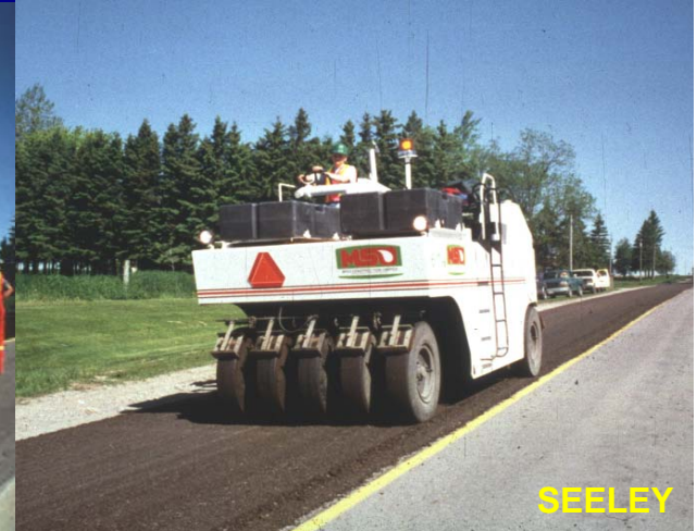
COMPACTION COMPLETED WITH LARGE RUBBER TIRED ROLLER
