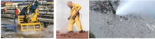
High pressure water blasting
