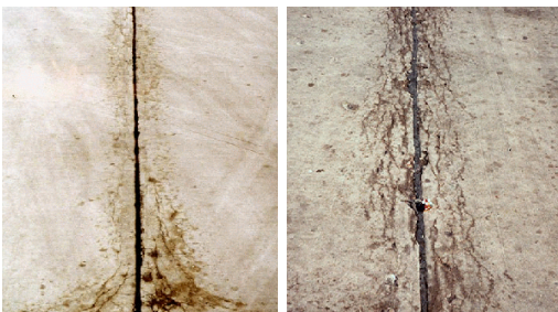
“D” Cracking
