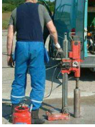
Coring is an excellent technique for preparing patch repairs
