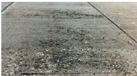
Scaling/Spaling
