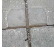
Cored corners of patch repairs
