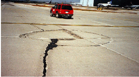
Corner Cracking (M)
