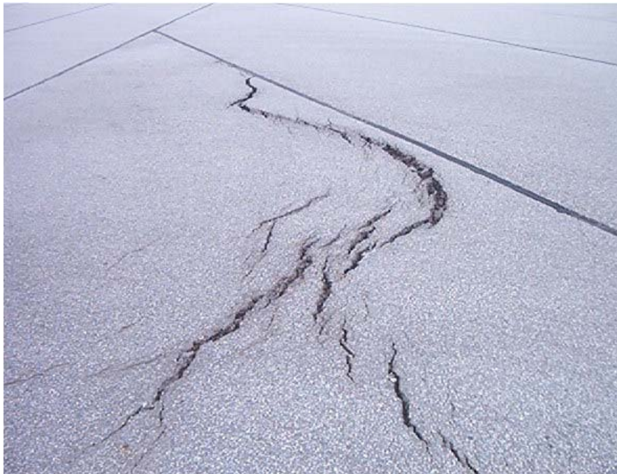
Asphalt slippage & shoving over PCC
