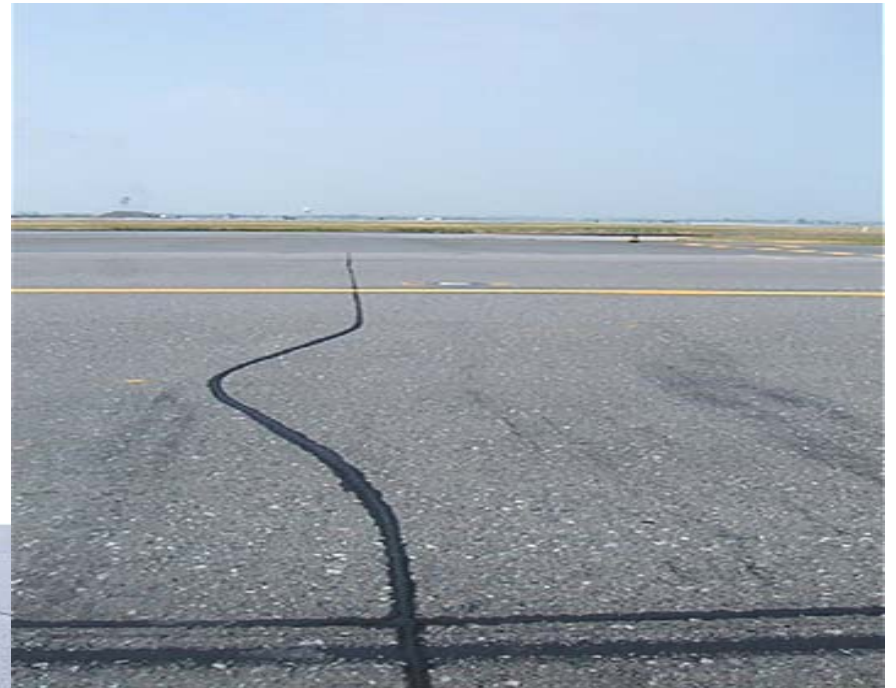
Asphalt Shoving at reflection joint on a taxiway
