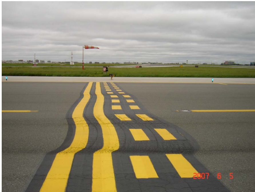
Pavement shoved at runway holdline position
