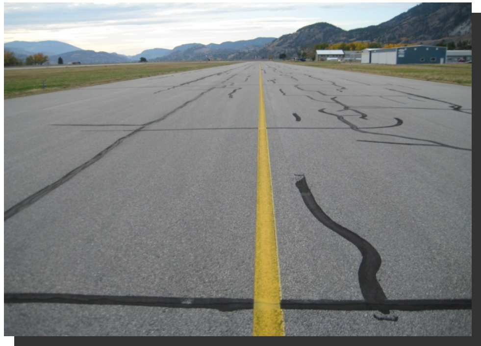
Stand-alone HIR surface – taxiway A at Penticton airport, completed 1994, as at October 2011 (17 years)
