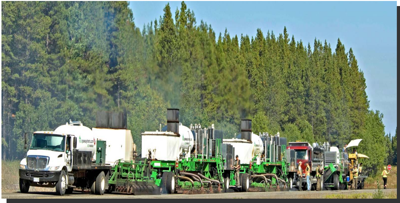
ARC Ecopaver 400 (2 stage) working on a BC highway project
