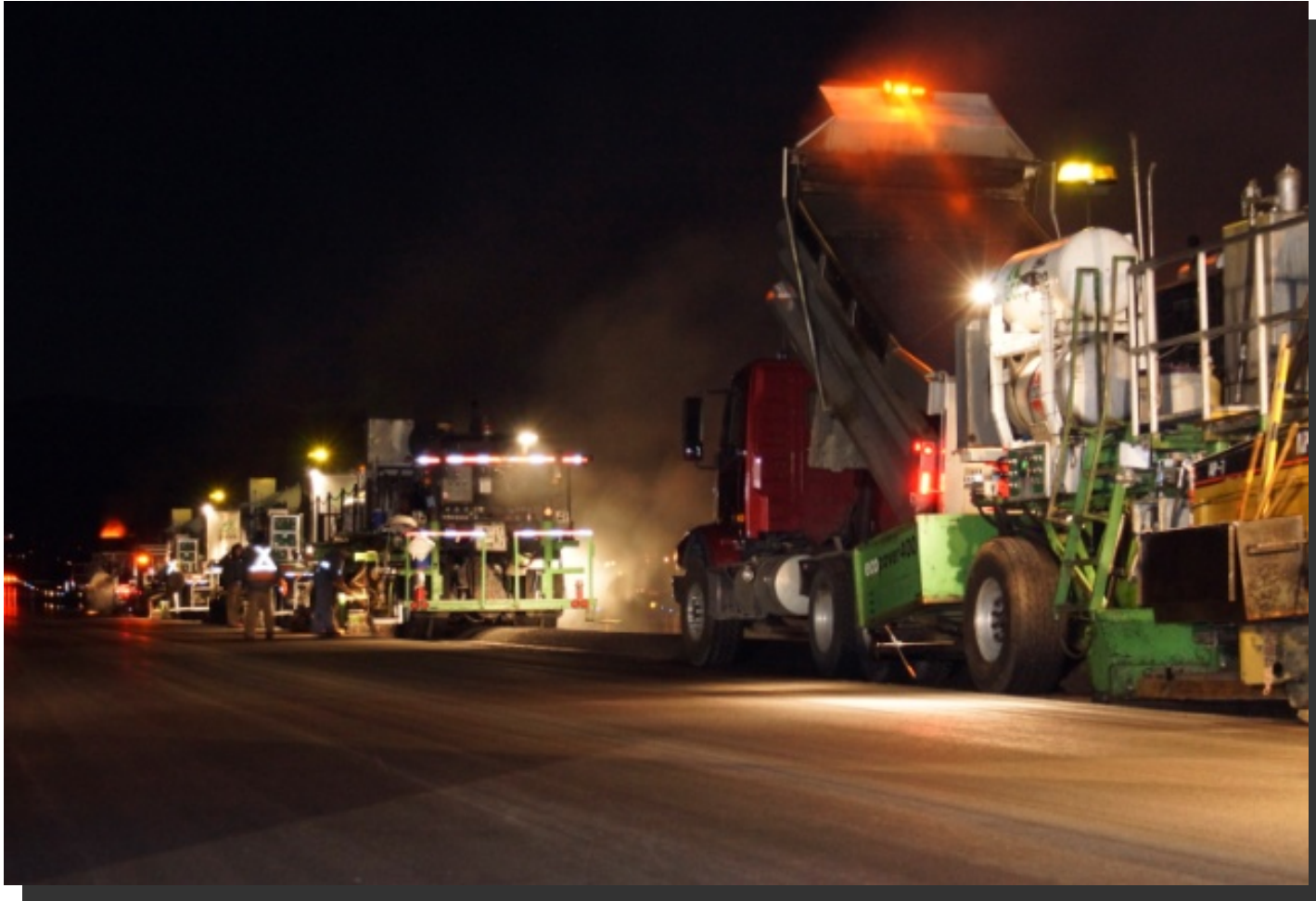
ARC HIR train from back of paver
