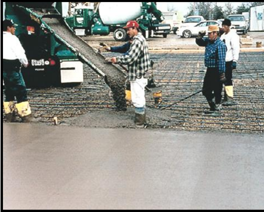
FLOWABLE CONCRETE IS PLACED
