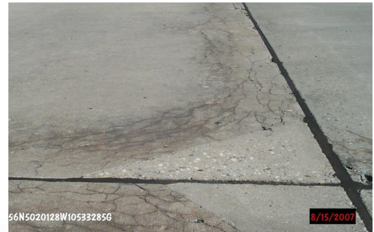
Durability cracking
