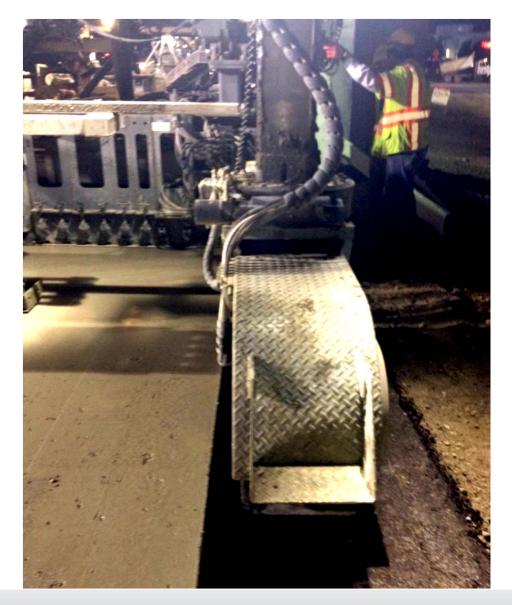
Rear Crawler Track Moved within Inches of the New Slab <u>On the Fly</u> Using "Smart Leg" Technology!
