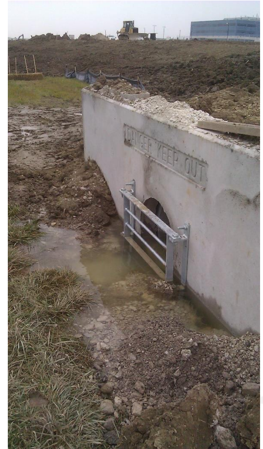
Connecting storm pipe to headwall
