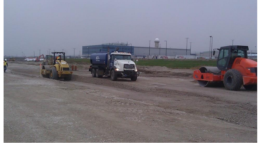
Applying water to obtain adequate moisture level
