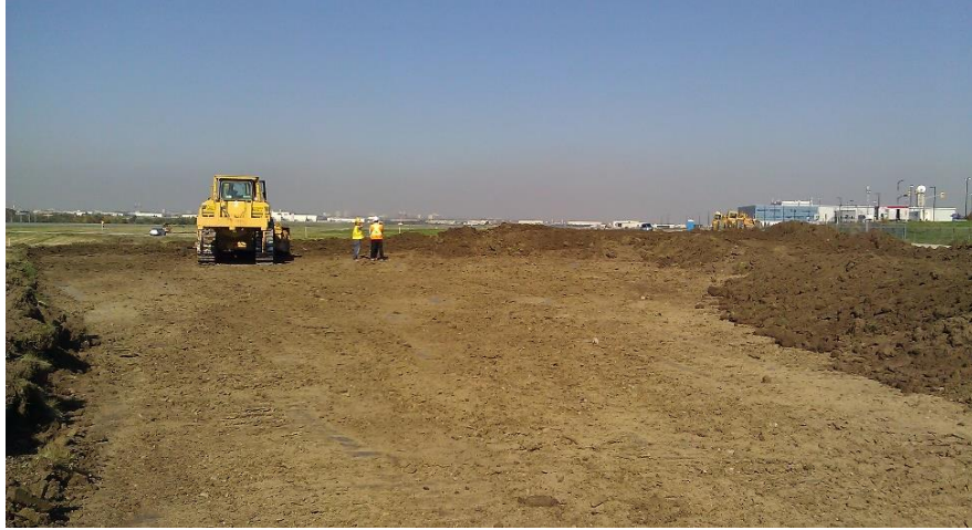
Stripping topsoil
