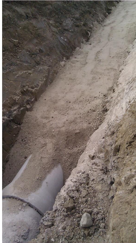
Laying down storm pipe and backfill with granular
