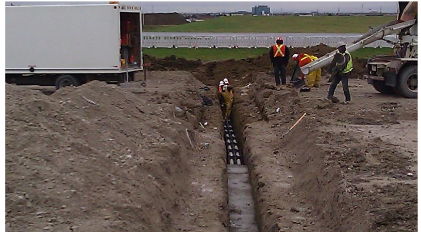
Concrete encased power duct bank crossing proposed taxiway alignment
