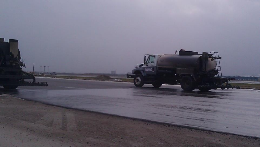
Applying tack coat and echelon paving surface course asphalt layer
