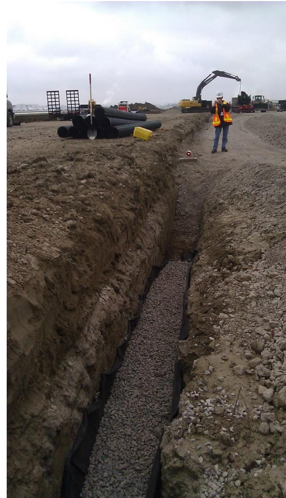
Backfilling with clear stones and wrapping around with geotextile
