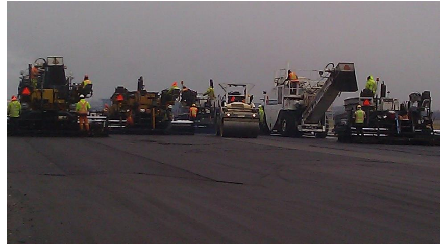
Applying tack coat and echelon paving surface course asphalt layer
