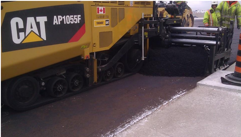
Applying prime coat prior to placing 1 st base course asphalt layer
