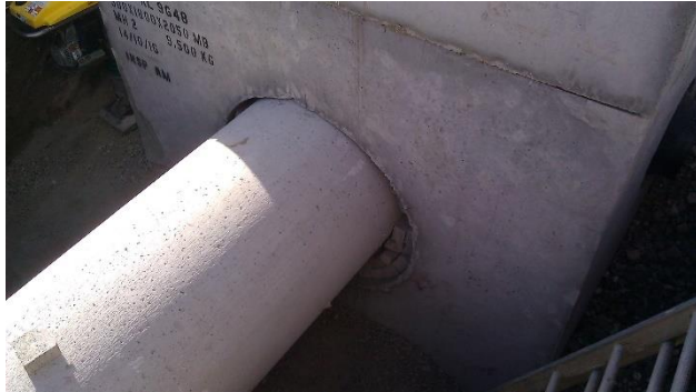
Connecting storm pipe to a catch basin
