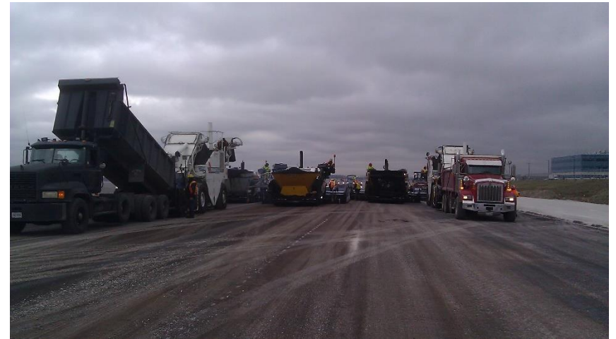
Echelon paving 1 st base course asphalt to eliminate longitudinal cold joint on the main taxiway. Shuttle buggy to reduce the possibility of segregation
