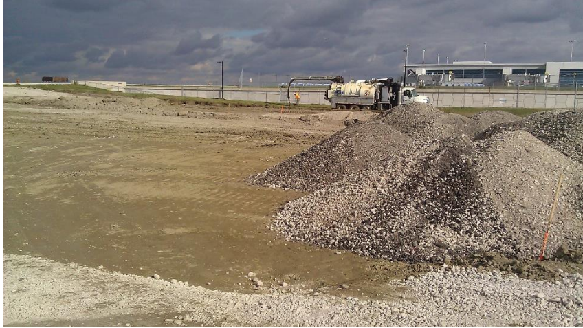
Placing recycled concrete aggregate as granular subbase material
