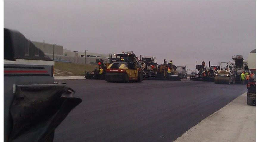
Applying tack coat and echelon paving 2 nd base course asphalt
