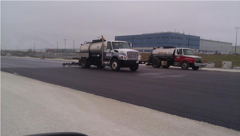
Applying tack coat and echelon paving 2 nd base course asphalt
