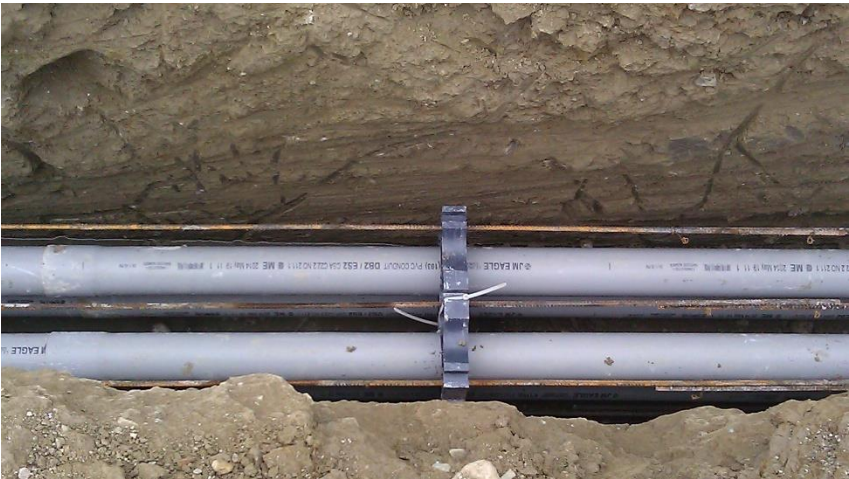
Concrete encased power duct bank crossing proposed taxiway alignment
