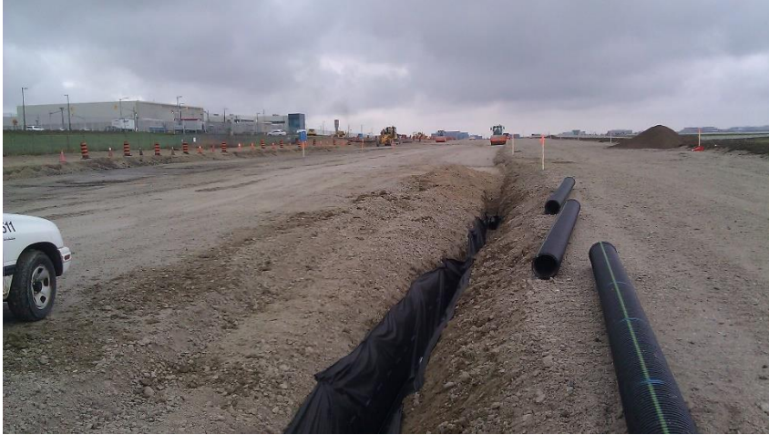
Laying down subdrain pipe
