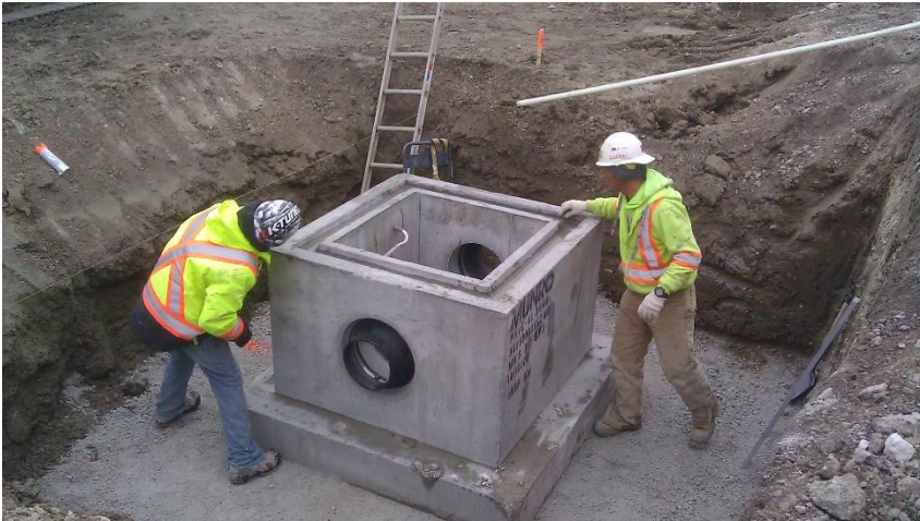
Laying down subdrain manhole
