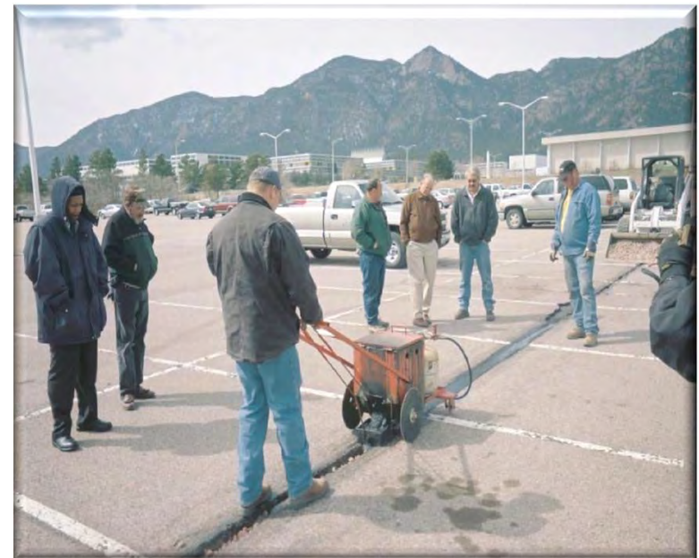
Using a mastic applicator with attached squeegee to fill large cracks.
