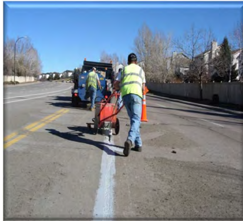
Installing Gray Mastic into longitudinal concrete joint.
