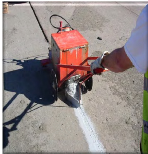
Using a V shaped metal squeegee to install Gray Mastic into smaller concrete joints.
