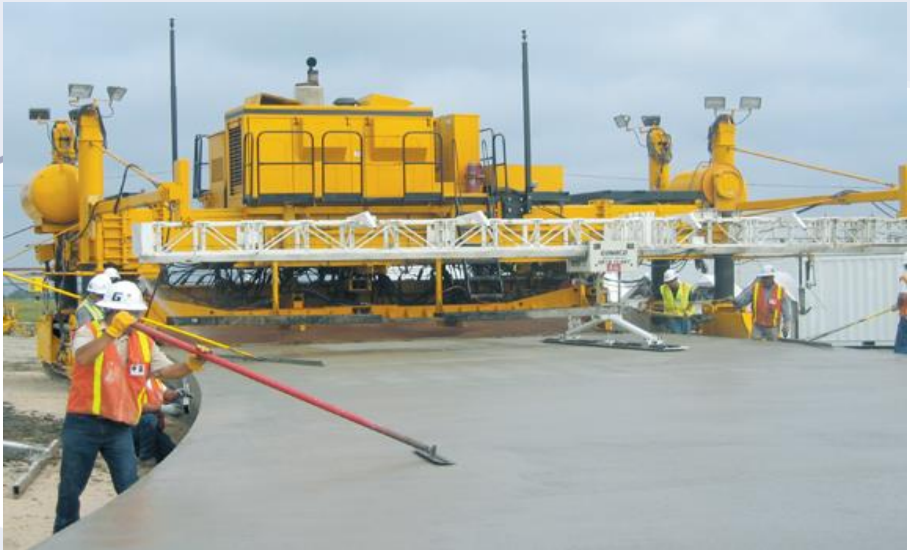
Stringless control of thick airport paving.
