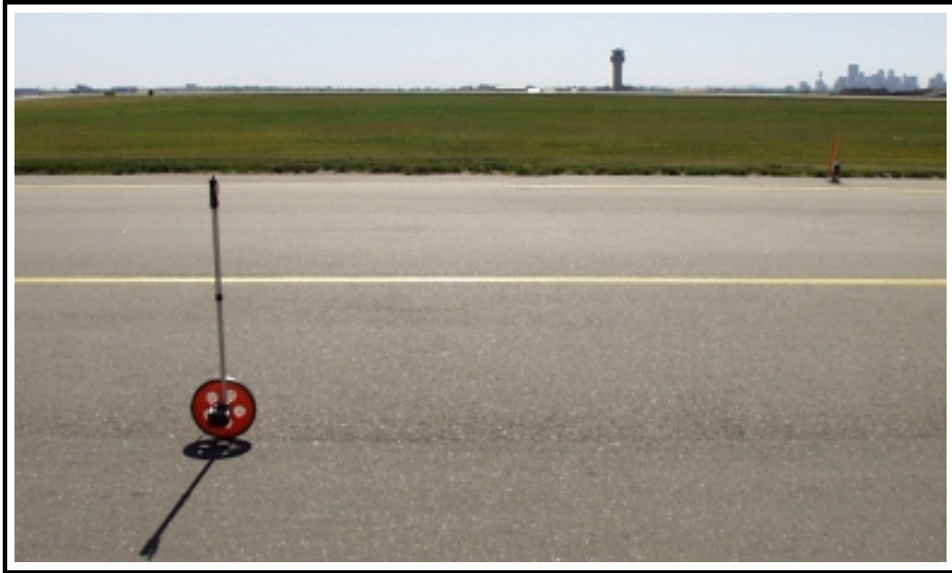
Photo 5 Low severity ravelling/weathering along longitudinal joint in PG Test Section - September 2000
