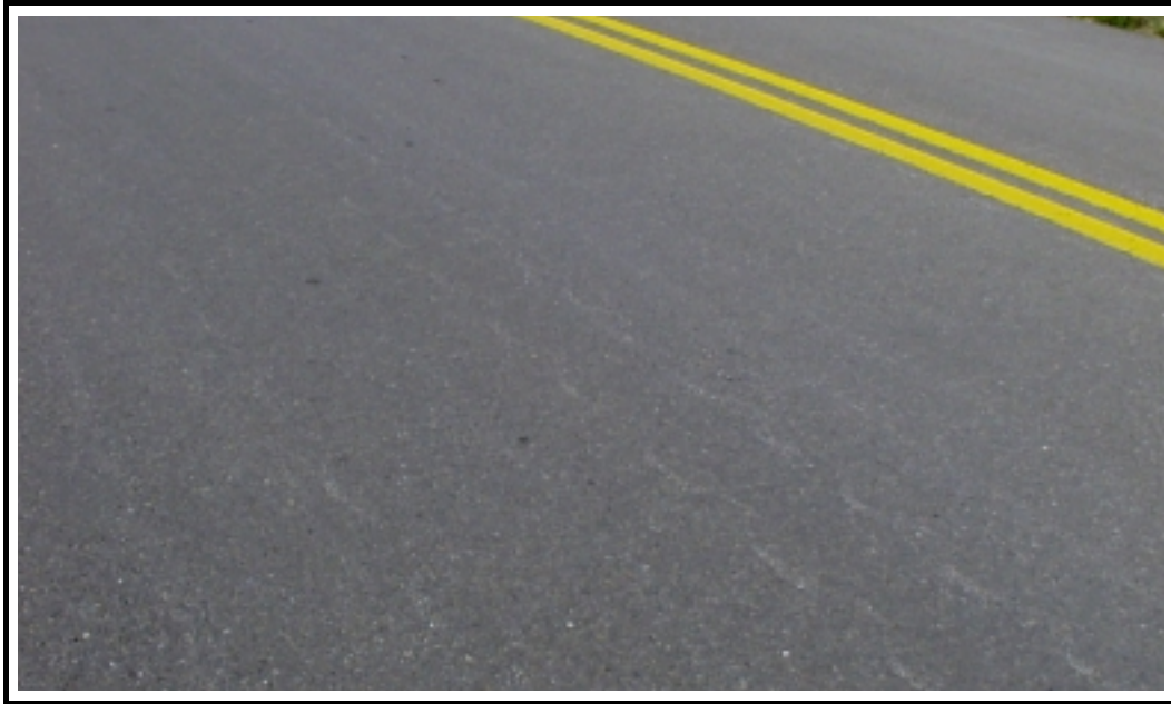
Photo 13 “Broom Marks” in Control Section - September 2000
