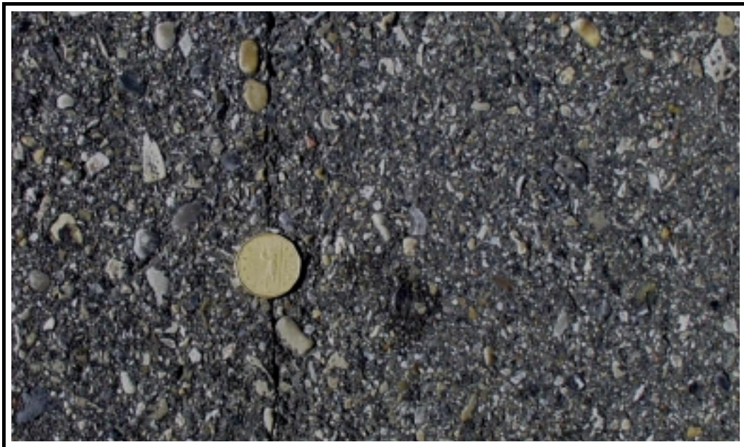
Photo 10 Close-up of hairline crack at saw cut longitudinal joint in PG Test Section (~2+110) (also represents Control Section) September 2000
