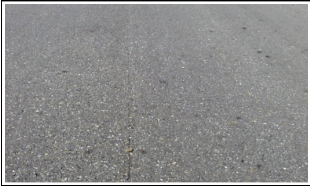
Photo 9 Hairline crack at saw cut longitudinal joint in PG Test Section (~2+110) (also represents Control Section) - September 2000
