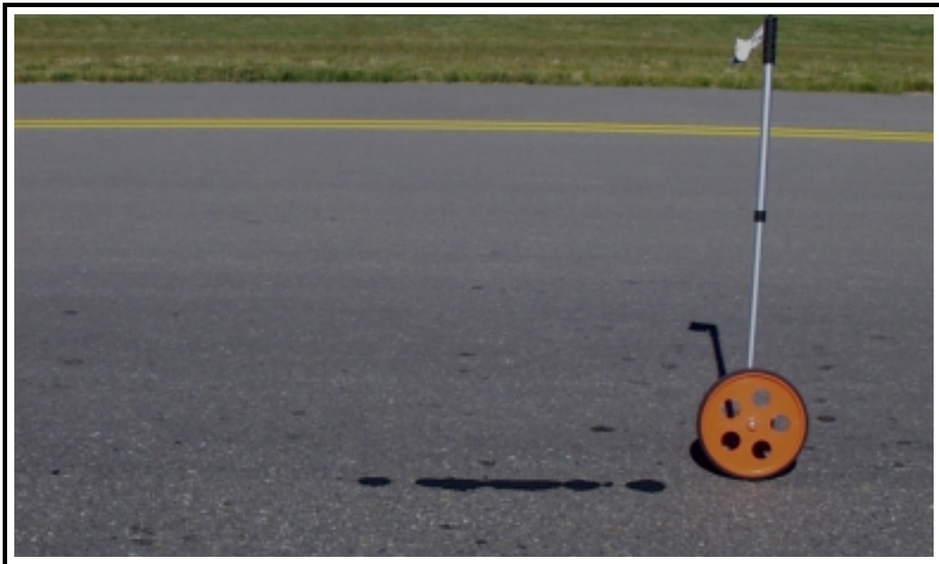
Photo 8 Minor bleeding along longitudinal joint in PG Test Section September 2000
