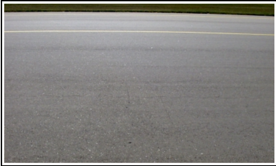
Photo 7 Example of screed mark in PG Test Section (also represents screed marks in Control Section) - September 2000
