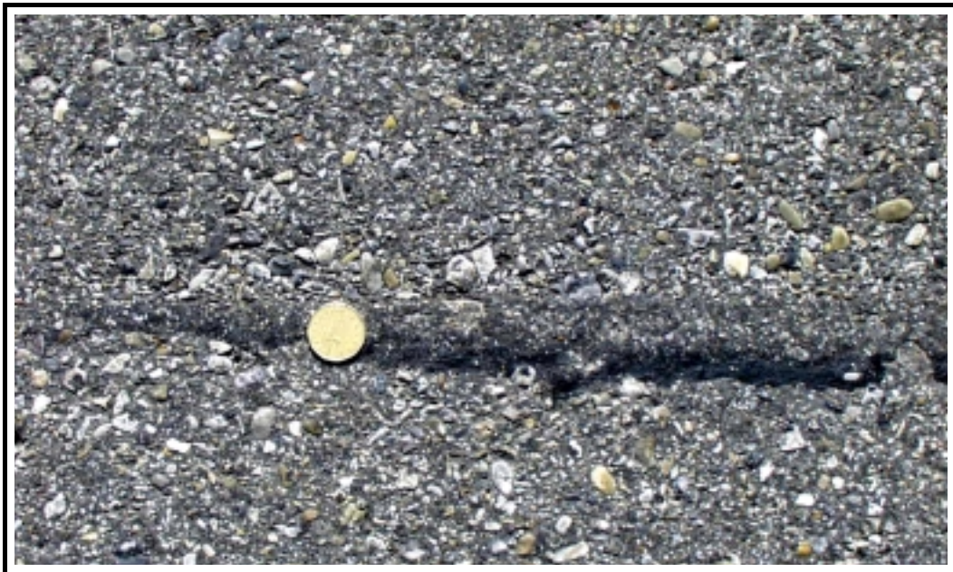
Photo 14 Minor bleeding at saw cut longitudinal joint in Control Section September 2000
