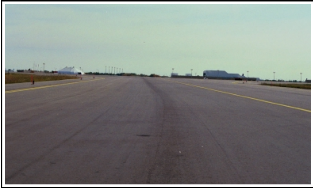
Photo 3 Low severity ravelling/weathering along longitudinal joint in PG Test Section - September 1999
