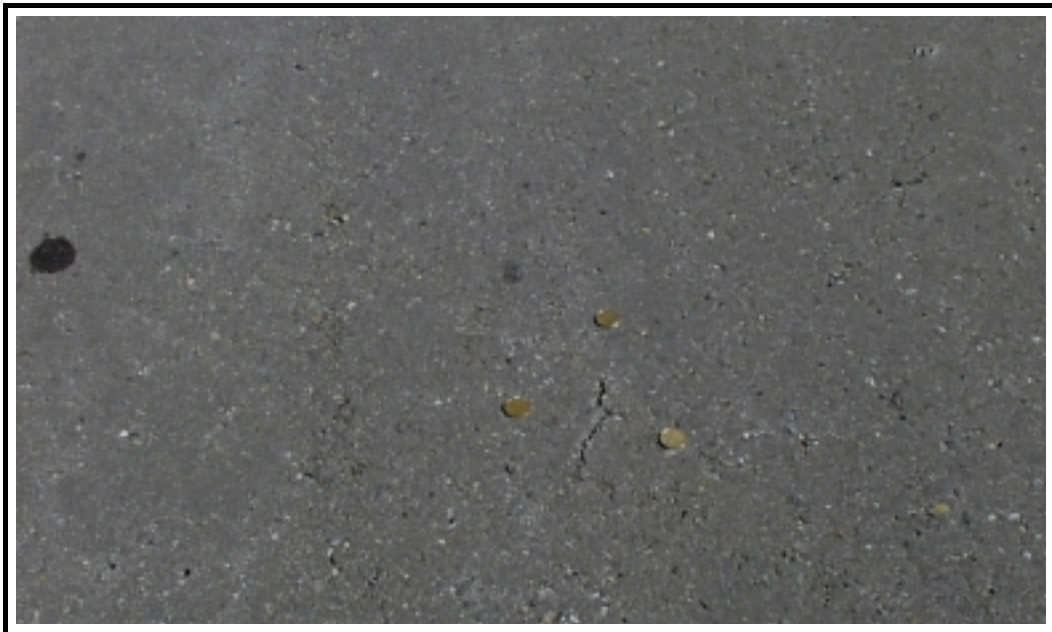
Photo 2 Very minor crack in PG Binder Test Section (~2+050) - September 2000
