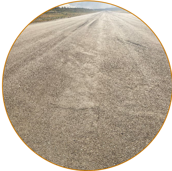
Well Graded with Recent 40mm Thick Overlay
