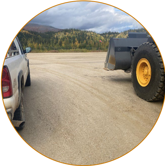
Transverse Slopes Draining Surface
