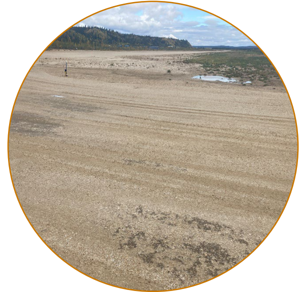
Low Severity Rutting / Tire Impressions
