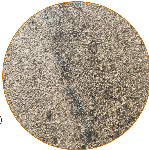
Tight, Compact Surface with Minimal Segregation
