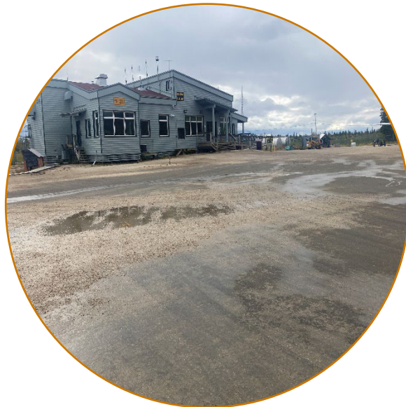
Shallow Depressions between EK35 Dust Suppressant Patches
