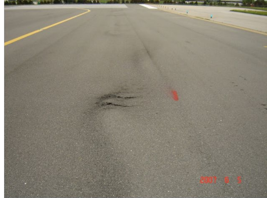
Shoving in asphalt due to heavy braking of fully loaded aircraft
