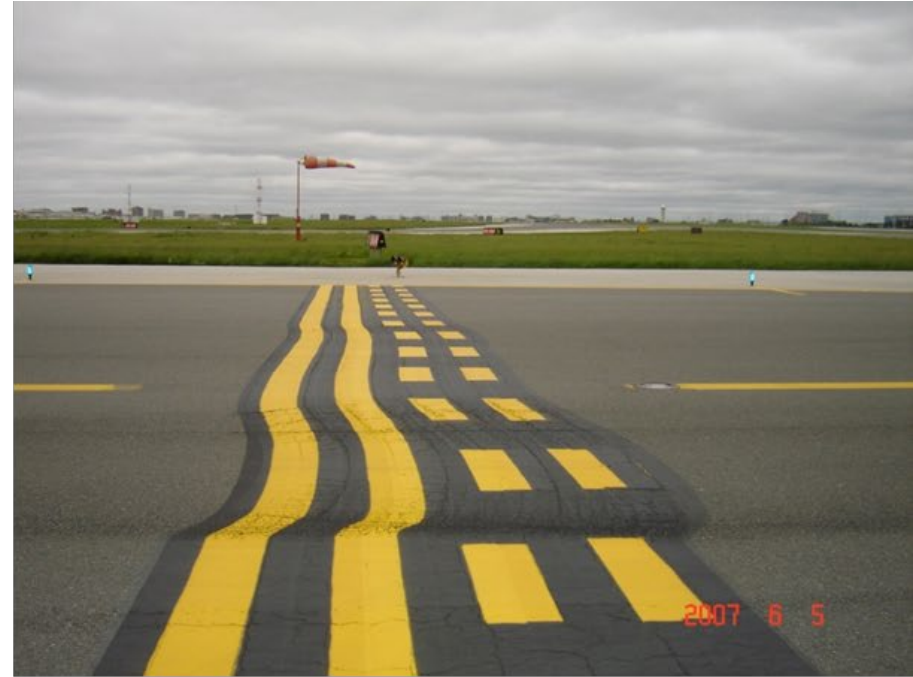
Pavement shoved at the hold line position
