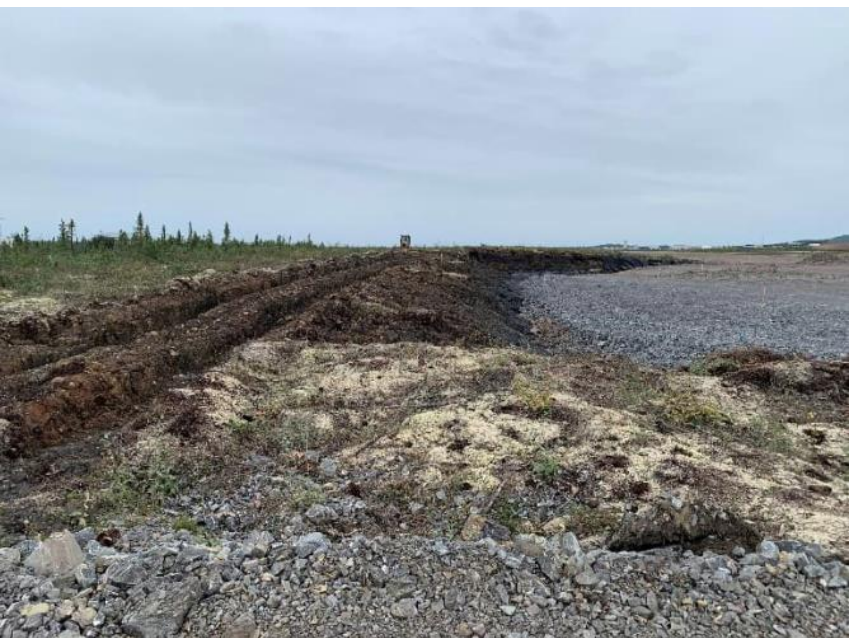
Sub excavation – Runway 24 aircraft turning pad area
