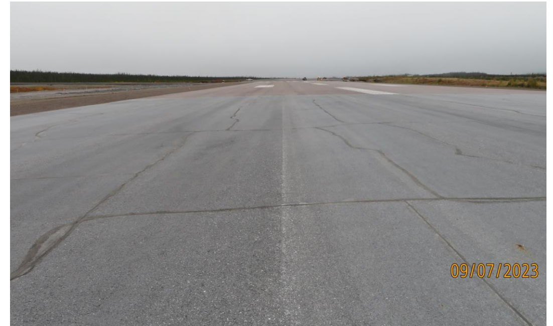
Runway 06-24 Sinkhole Repair Area
