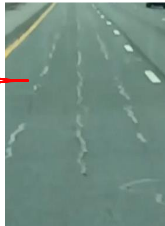
Premature Crack
