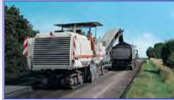
Pavement Milling
