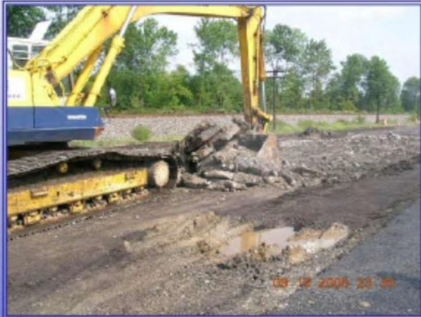
Asphalt Pavement Removal
