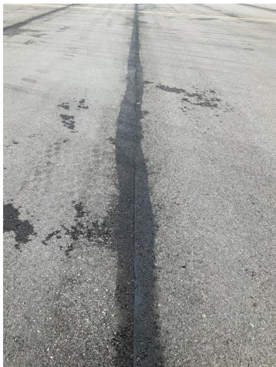
Longitudinal cracks (construction joints)
