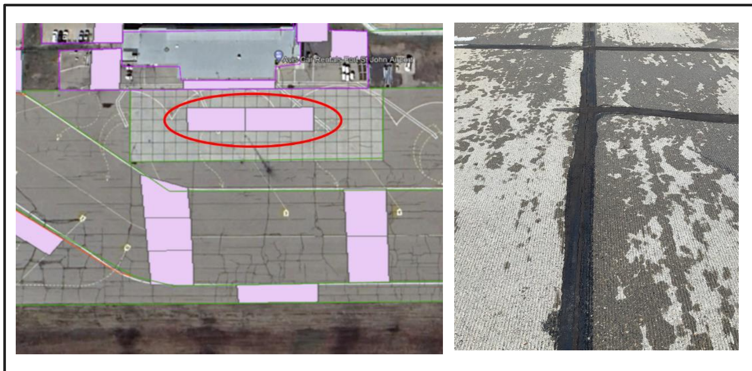
Joint sealant in moderate condition
