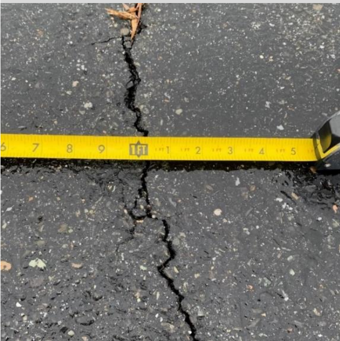
Visual Pavement Condition Survey
