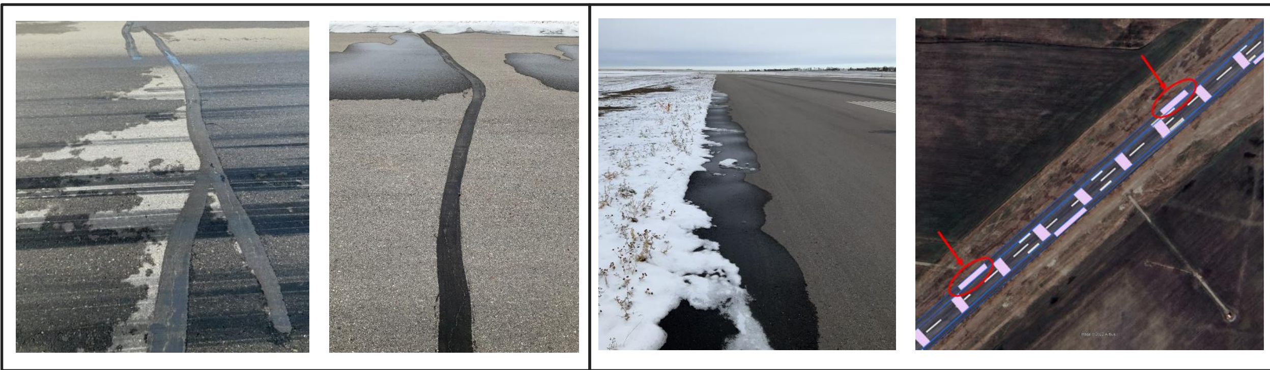
Transverse Cracking
