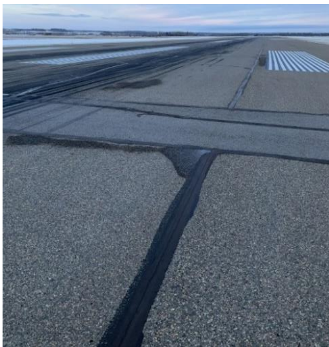
Crack seals and patching mostly in good condition
