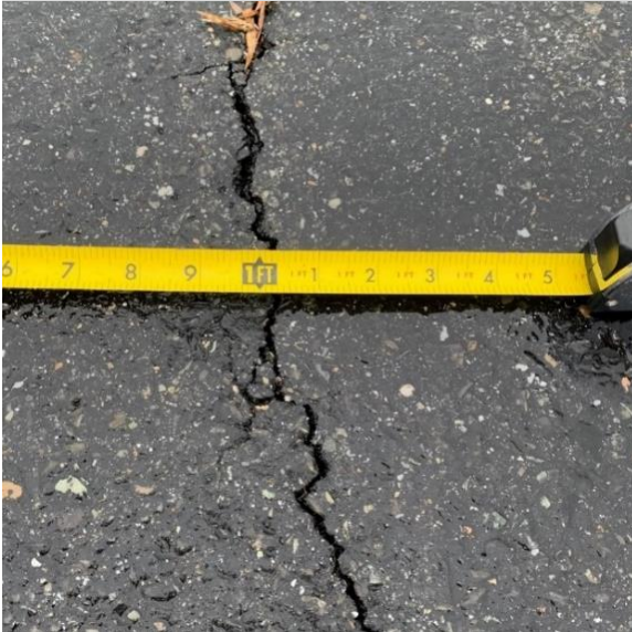
Visual Pavement Condition Survey
