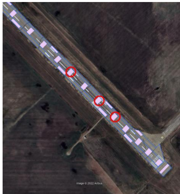
Isolated spots with rutting and spalling
