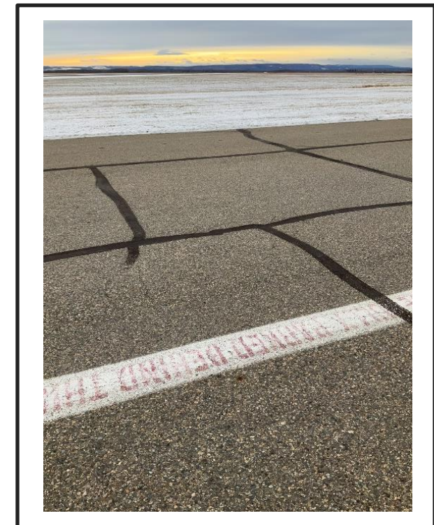
Transverse Cracking
