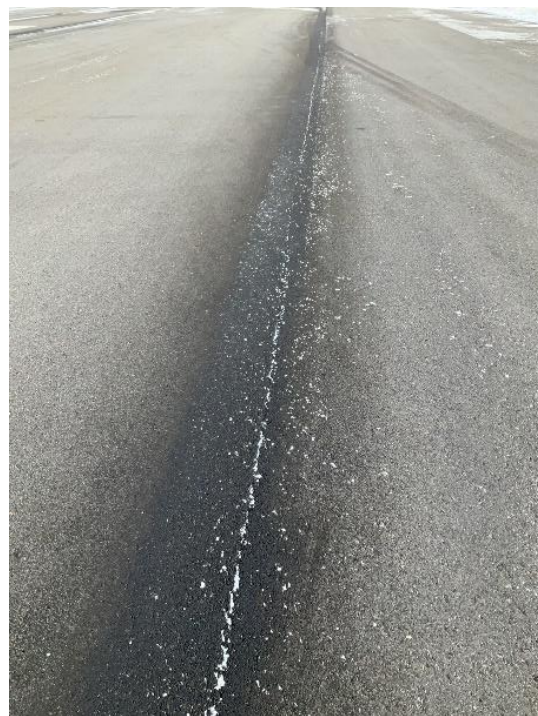
Longitudinal cracks (construction joints)
