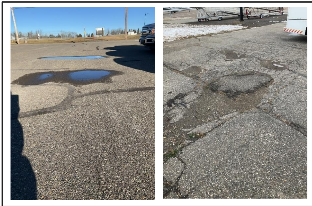
Pavement distortions
